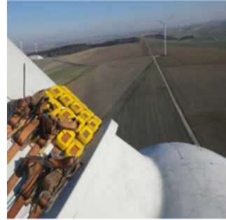
Rotor imbalance adjustment
