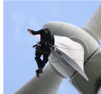
Rotor blade inspection
