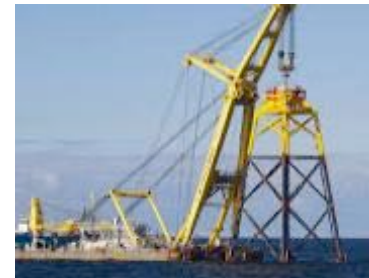
Pile and Jacket installation supervision
