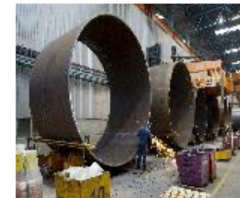
Pile and Jacket construction supervision
