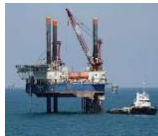
Crane and barge inspection and acceptance
