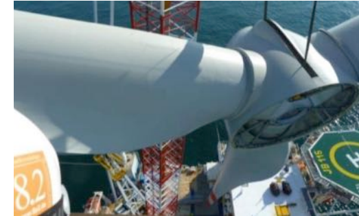
Mechanical installation supervision
